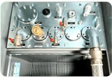
V-H from the rear - Overfill protection, overpressure vacuum valve & larger flange/ inspection hatch
